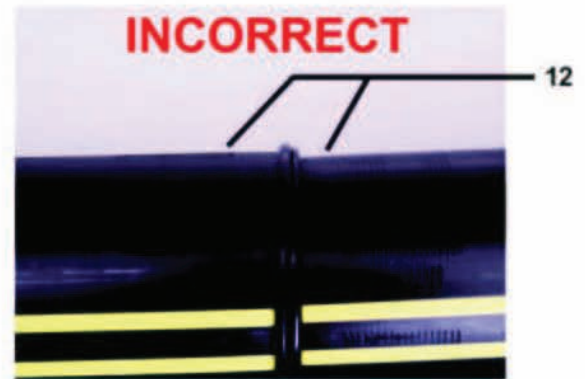
12. Improper "High-Low" alignment
